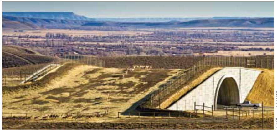
Pronghorn locate and use newly-constructed highway overpasses that safeguard wildlife and motorists on US 191 at Trapper's Point, Wyoming (Fall 2012).
