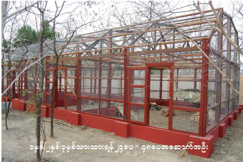
New juvenile rearing facilities for star tortoises at Minsontaung WS. Designed to be both theft and predator (rat) proof, this is a model enclosure that can be used in other locations.
