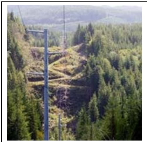
Photo 4: power line passing through a forest with trees cleared on either side to prevent wires from touching (BPA transmission Line, Olympic Peninsula, Oregon, USA. 2008)
